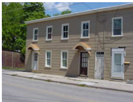
Future home of Olde Getty Place's community room
